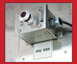
When all else fails, hit the red button to shut down the rig.
